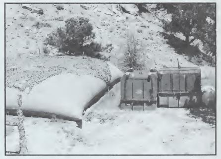
Another collection system provides water to this 50,000-gallon collapsible tank, where it is conveyed by a booster pump to a permanent storage tank located 2 miles away and 600 feet higher in elevation. The water is then distributed by gravity flow through approximately 7 miles of pipeline to four sets of troughs.
